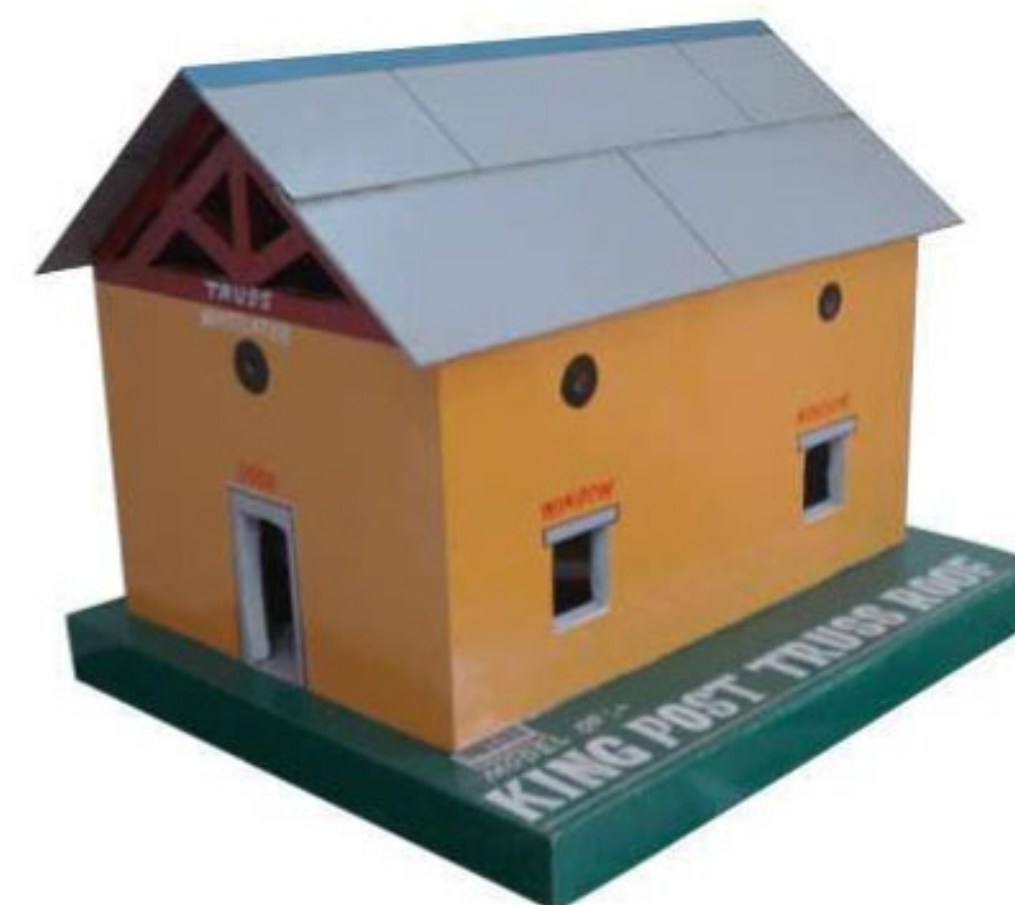
King Post Truss Roof
