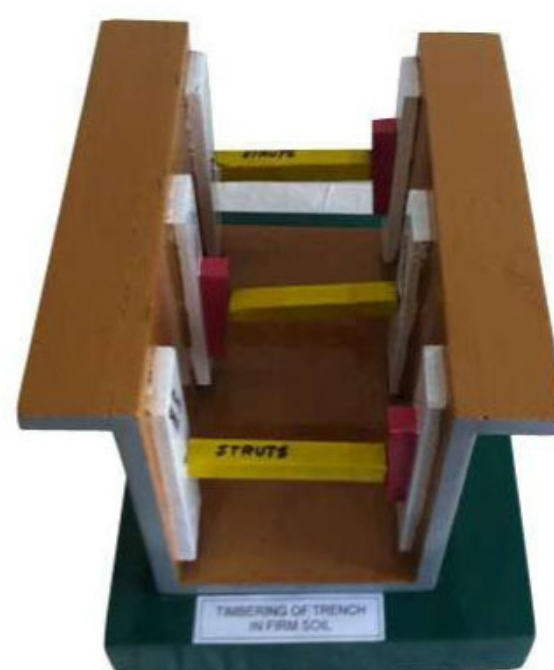
Timbering of trench in firm soil
