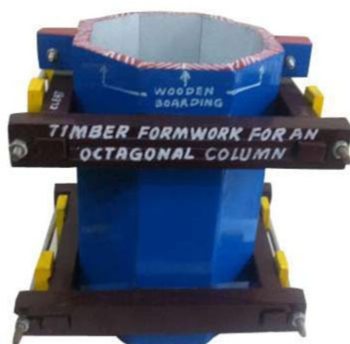
Timber form work for octagonal Column
