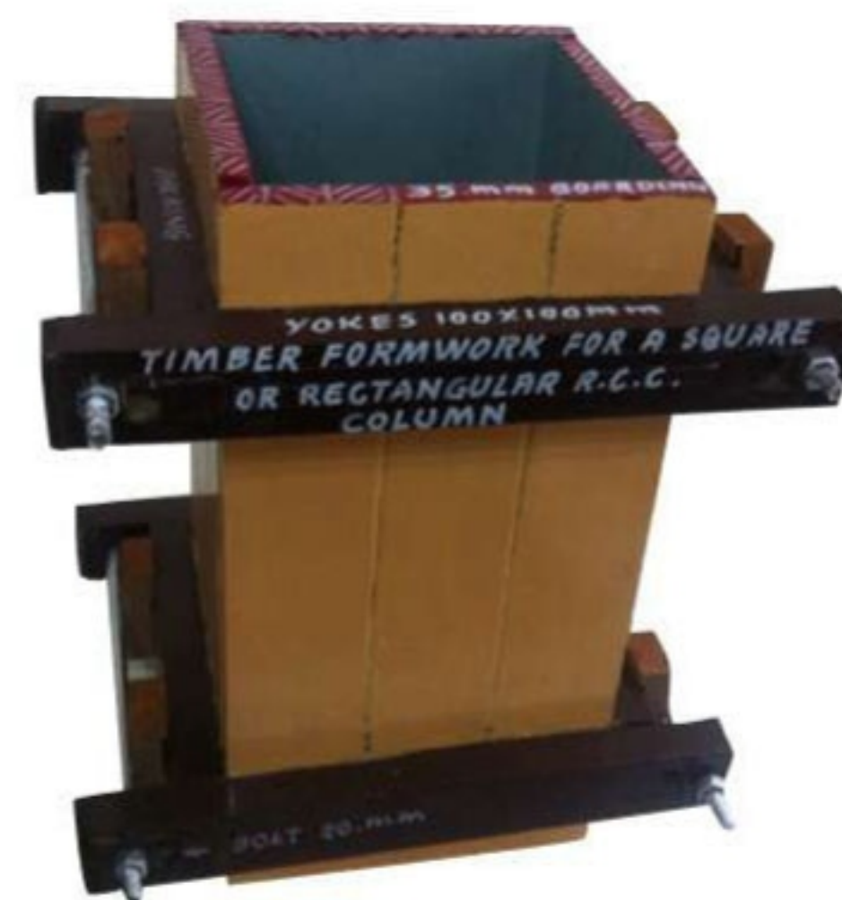
Timber form work for square Or Rectangular column
